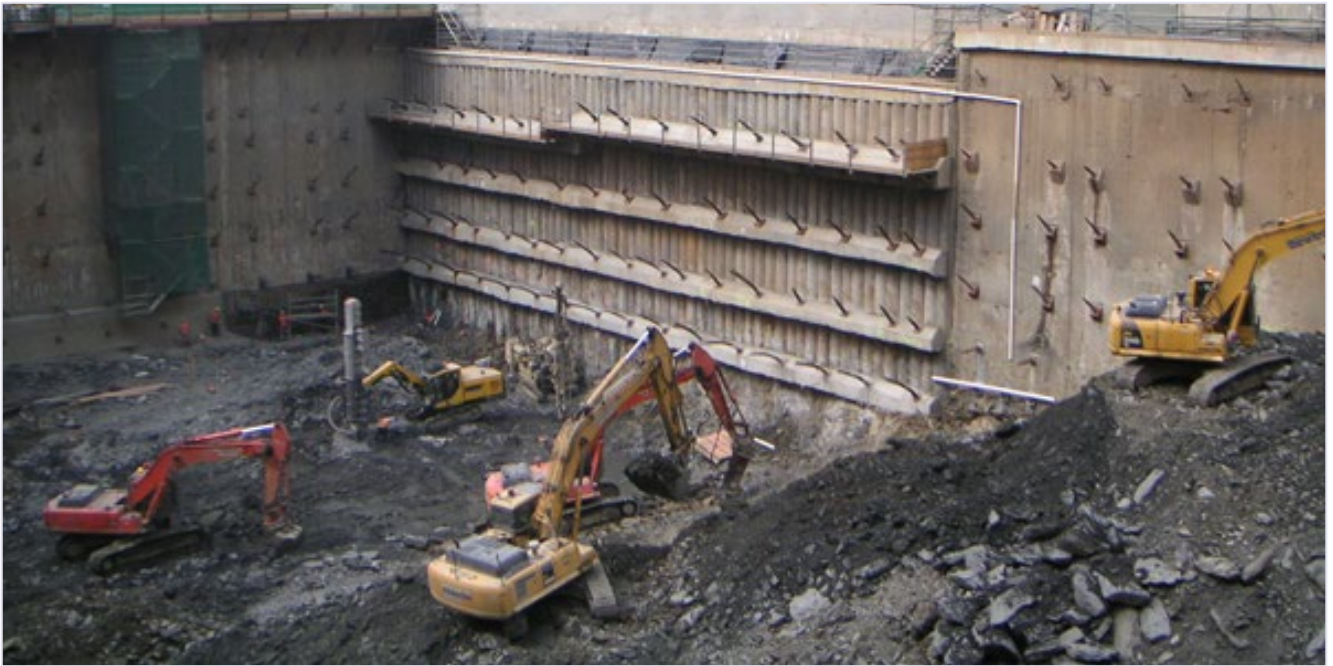
Diagram 19.19: Secant Piles in a Shaft and a D-Wall in an Underground Station for Avoiding Groundwater Influx
